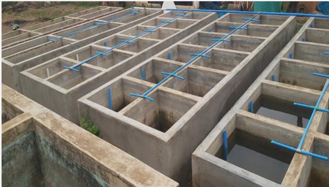
Figure 10 Fish concrete tanks (Photo by author)
