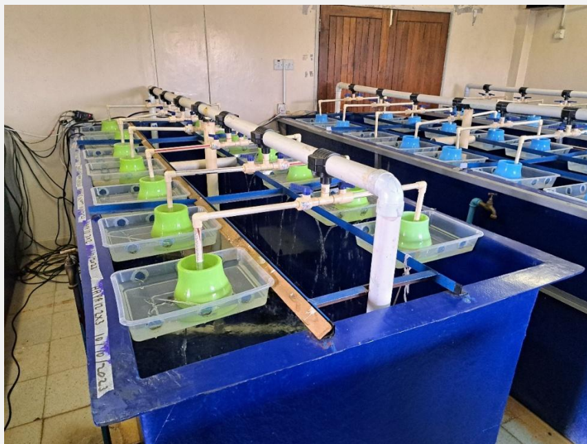
Figure 14 Tilapia fish hatchery utilising a Recirculatory Aquaculture System (RAS) at the National Aquaculture Research Development Centre (NARDC) (Source: Chad Kancheya)
