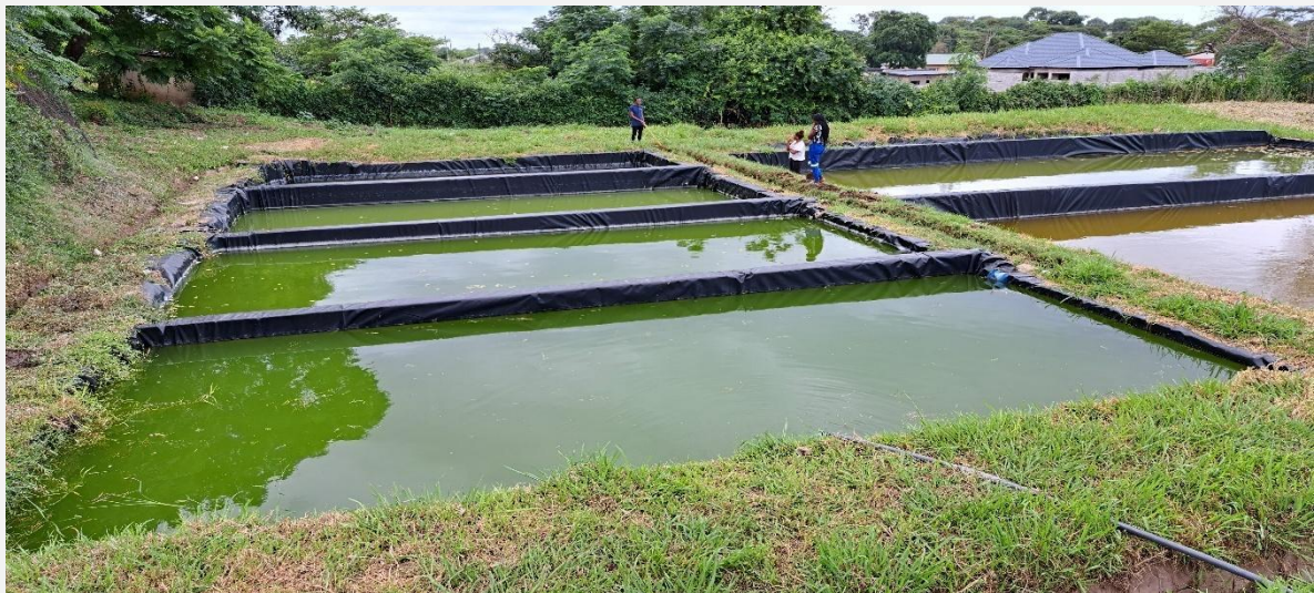
Figure 11 Concrete tanks installed with a dam liner to improve water retention at Chilanga Aquaculture Research Station in Chilanga district (Source: Chad Kancheya)
