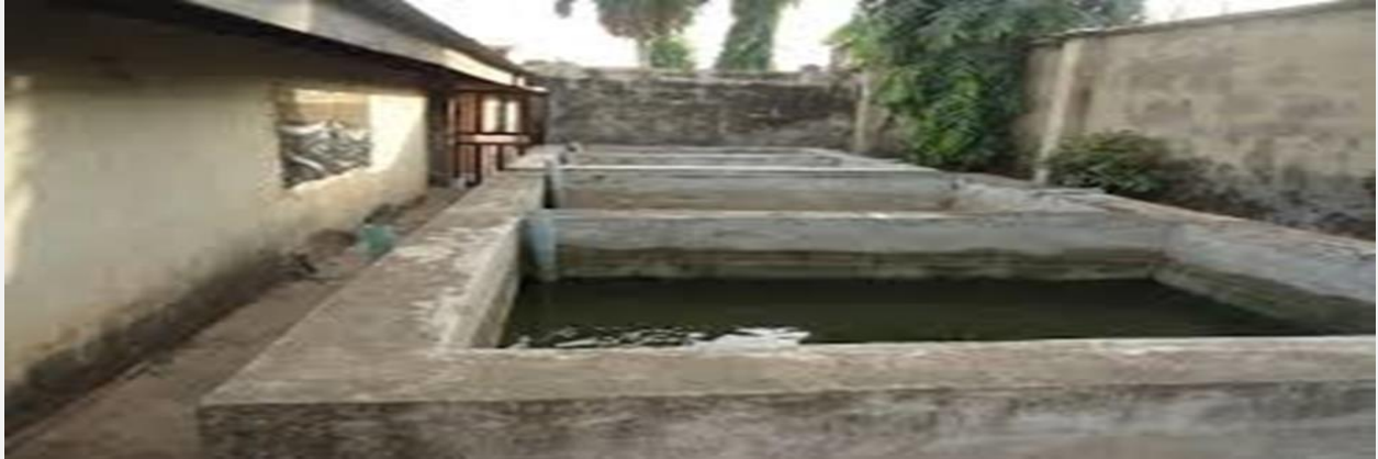
Figure 4 An intensive, concrete tank aquaculture system
