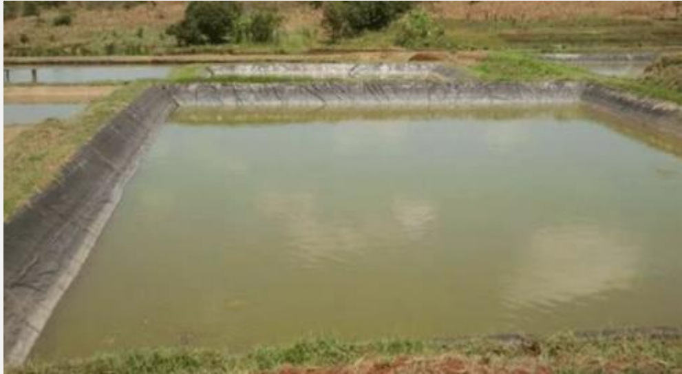
Figure 6 Tarpaulin reinforced earthen pond
