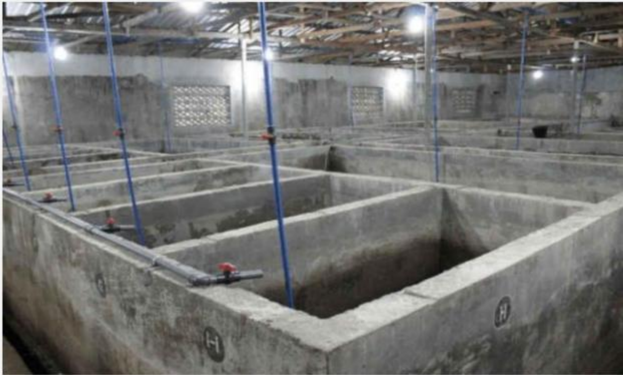
Plate 6 Concrete tanks built in an enclosed housing space to house fish; Source – Everlush.ng
