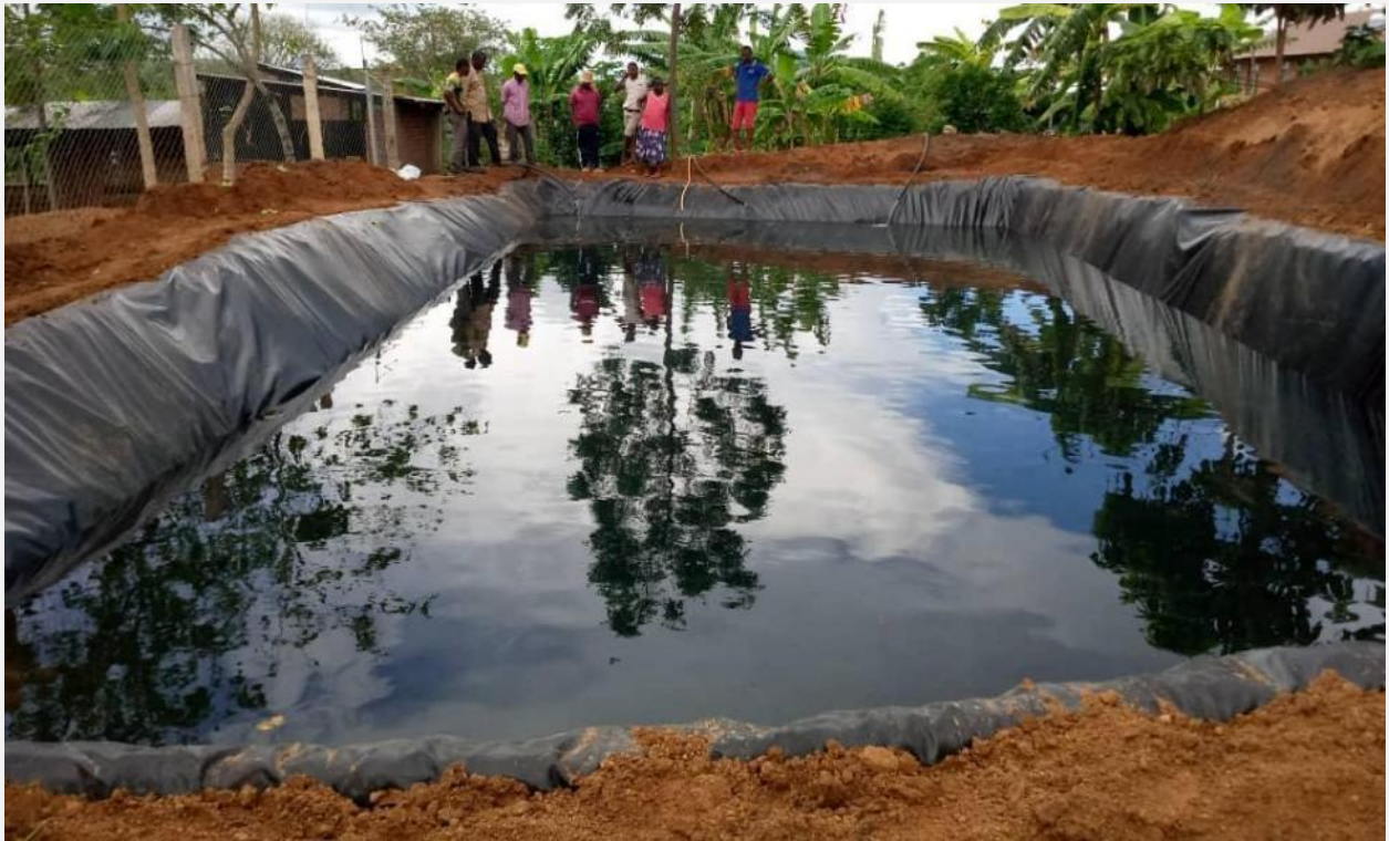
Plate 9 Photograph of tarpaulin pond set-up to house fish with tarpaulin material placed in a dug-out earthen space; Source – Everlush.ng
