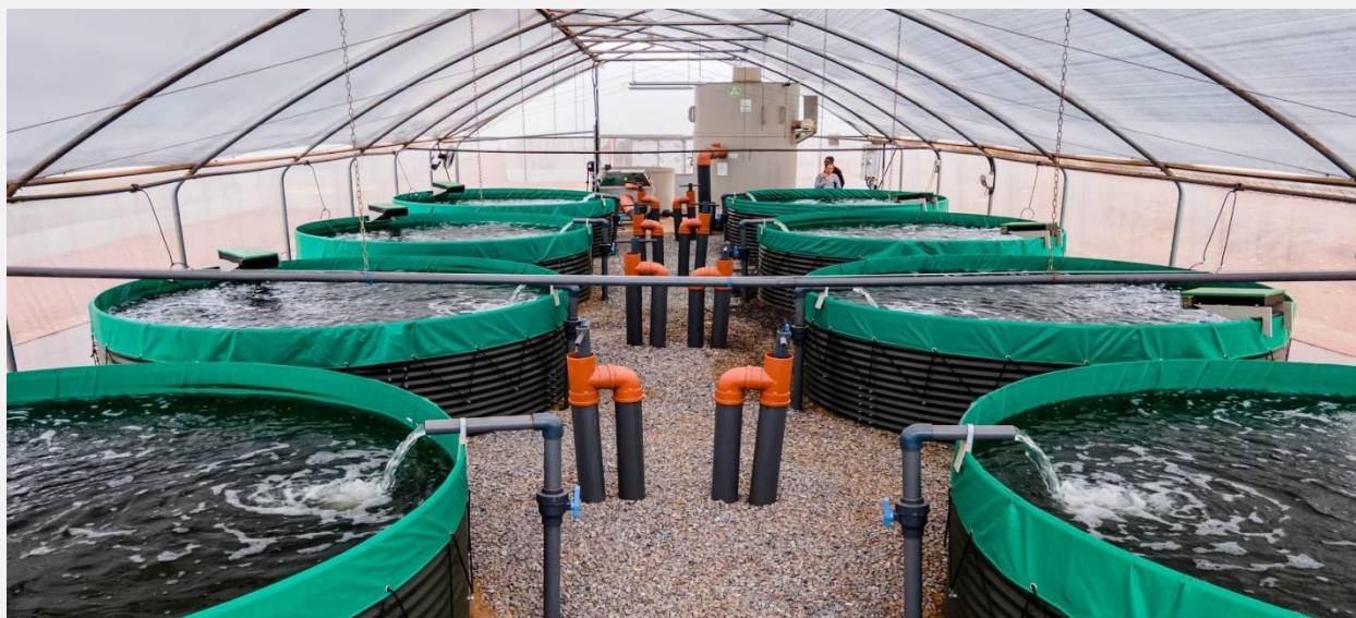
Figure 4 Circular tanks (Greenhouse RAS system with paddle-wheel aerator and biofilter), an example of an Intensive aquaculture system. National Aquaculture Training Centre, Amrahia, Accra. Source: https://www.agritopgh.com/project/national-aquaculture-centre/
