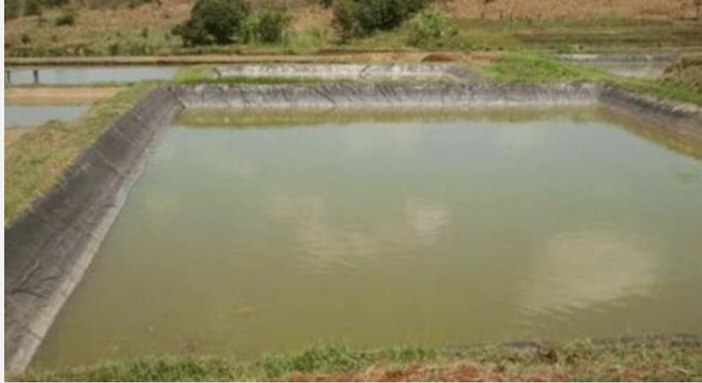
Figure 6 Tarpaulin-reinforced earthen pond
