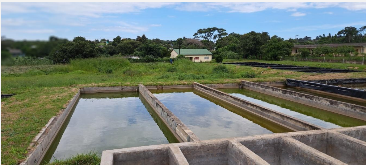
Figure 10 Concrete tanks constructed to culture fish at Chilanga Aquaculture Research Station in Chilanga district (Source: Chad Kancheja)
