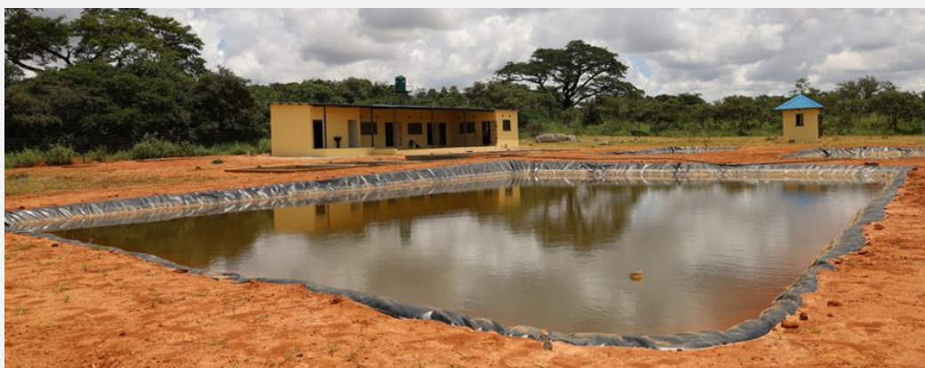
Figure 1 Pond-based system using dam liners (Source: WorldFish Centre/NRDC, 2019)
