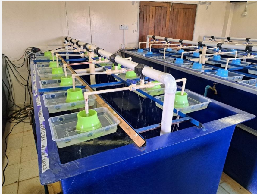
Figure 14 Tilapia fish hatchery utilising a Recirculatory Aquaculture System (RAS) at the National Aquaculture Research Development Centre (NARDC) (Source: Chad Kanchea)
